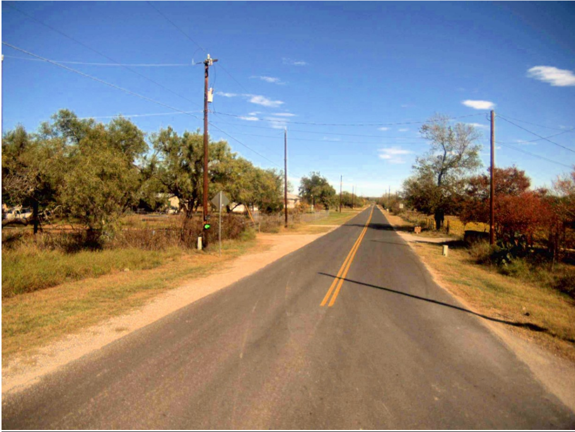
Sample image of pavement striping collected with MAC LRIS system
